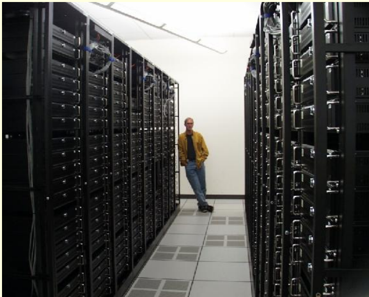
Google servers in a server farm
